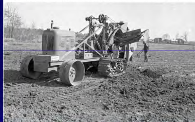
Laying subsurface drain tile with a machine. Shallow tiles and ditches were generally dug by hand. About four miles west of Dawson, Lac qui Parle County, circa 1905. (MHS photo)
