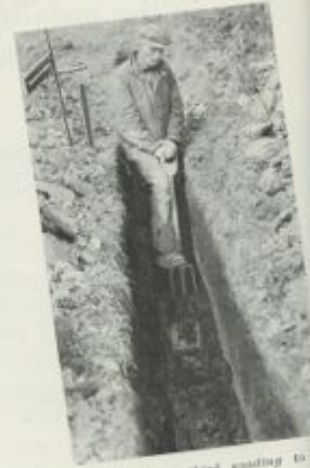
Digging the third spading to the right width and depth.
