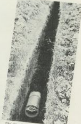
The line is all covered and the end tile plugged to keep out dirt and wa- ter.
