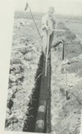
Grouping the bottom of the ditch to insure it is the right depth and the fall is uniform.
