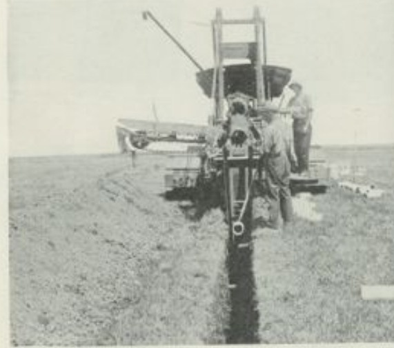
Digging the ditch by machinery. A terry grad, and a subsoiling aug. Do always lay the tile by hand—never by machinery.
