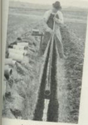
Laying the tile.
