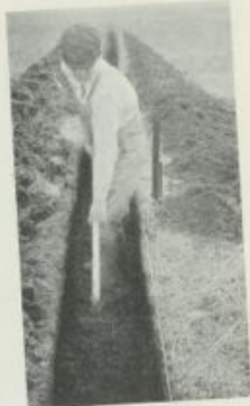
Cleaning out after the first spading and throwing the dirt back out by itself to one side of the ditch.
