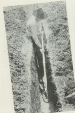
Cleaning and shaping the bottom ready to receive the tile.
